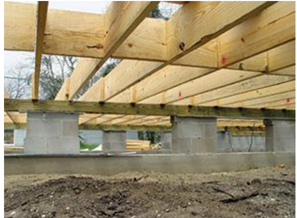
Figure 9: Pier and Beam Foundation
